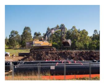
An excavator forms a stockpile as it digs a pipe trench
